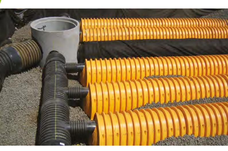
The unique Isolator Row is a water quality treatment device that's been independently NJCAT tested to eliminate over 80% of Total Suspended Solids (TSS). Isolator Row is built-in to ADS StormTech systems, helping to remove silt, metals, hydrocarbons, phosphorus and nitrogen, plus other surface water pollutants.
