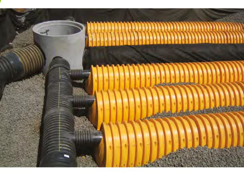
The difference is our unique Isolator Row. It's a water quality treatment device that's been independently NJCAT tested to eliminate >80% of Total Suspended Solids (TSS). Isolator Row is built-in to ADS StormTech systems, helping to remove silt, metals, hydrocarbons, phosphorus, nitrogen and other surface water pollutants.
