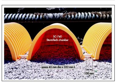
Figure 7 Spacing of chambers
