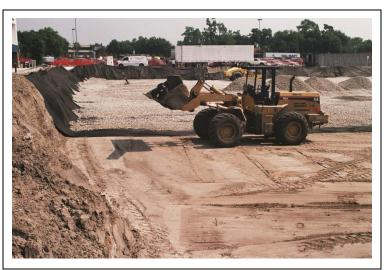
Figure 6 Installing foundation layer
